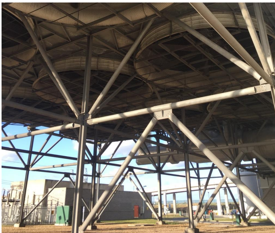
Plate: 3.10 RRRF Air Cooled Condensers
