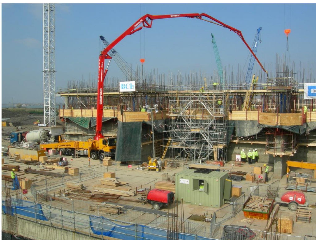
Plate 3.17: Typical bunker during a slip form operation
