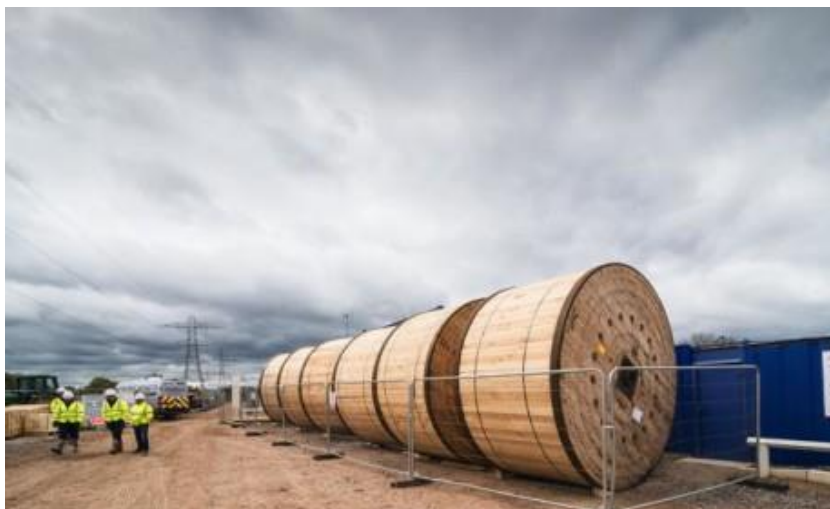
Plate 3.20: Example of 132kV Cable Drum Storage in Cable Route Temporary Construction Compound
